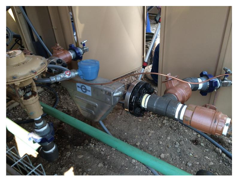
Figure IV.3-6. Coriolis oil flow meter.
