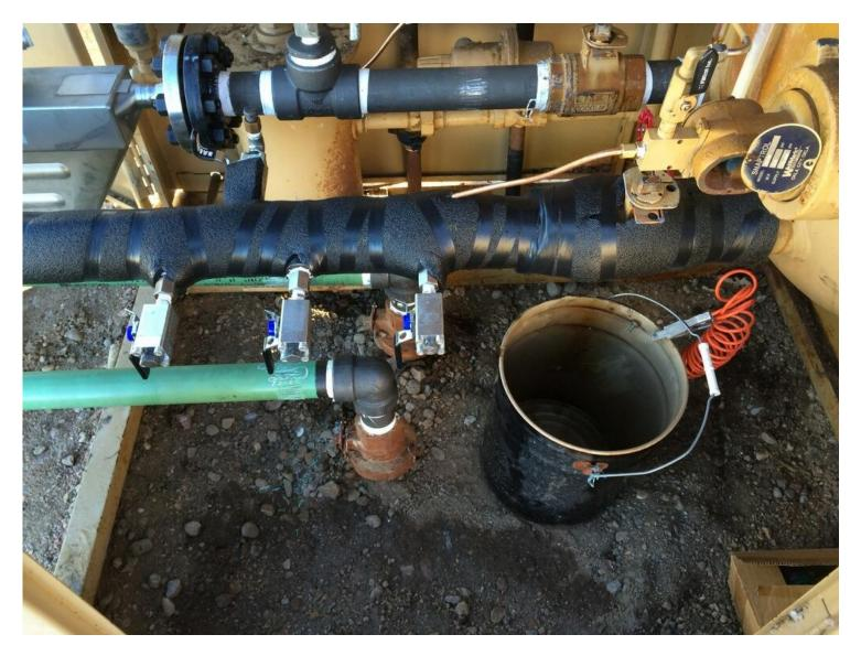
Figure IV.3-7. Pressurized condensate sample ports and oil box sight glass (upper right corner).
