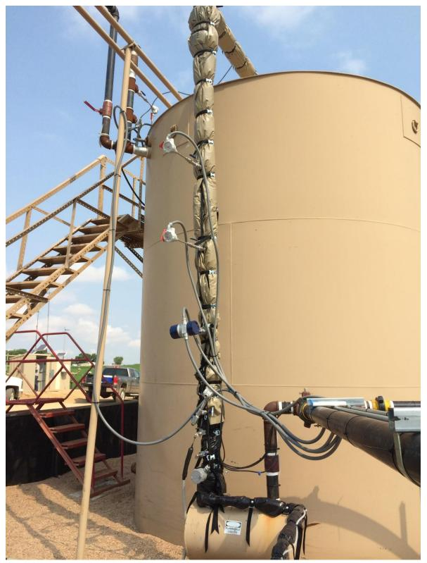
Figure IV.3-5. Condensate Storage Tanks with three gas flowmeters in insulated and heat-traced tank-to-burner pipeline. Gas sample collection port above knockout drum.
