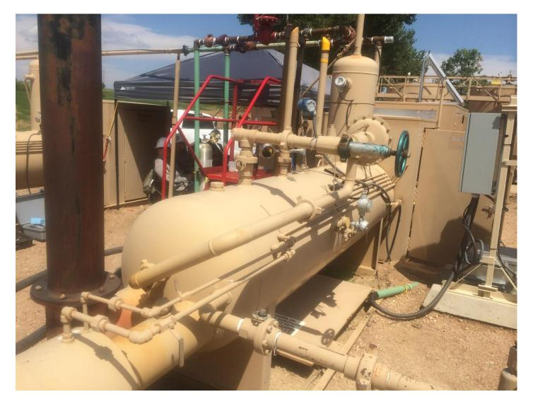
Figure IV.3-4. Test separator with back-pressure control regulator (red device at top of picture).
