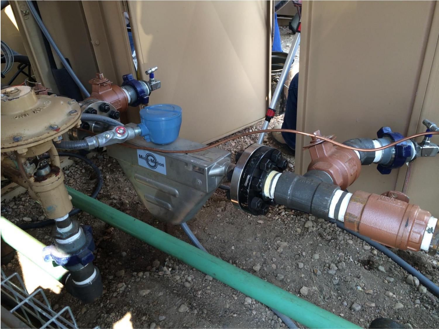
Figure IV.3-6. Coriolis oil flow meter.
