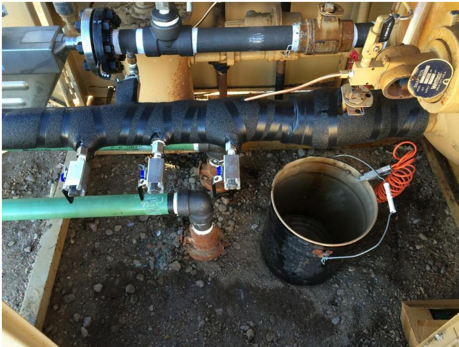
Figure IV.3-7. Pressurized condensate sample ports and oil box sight glass (upper right corner).
