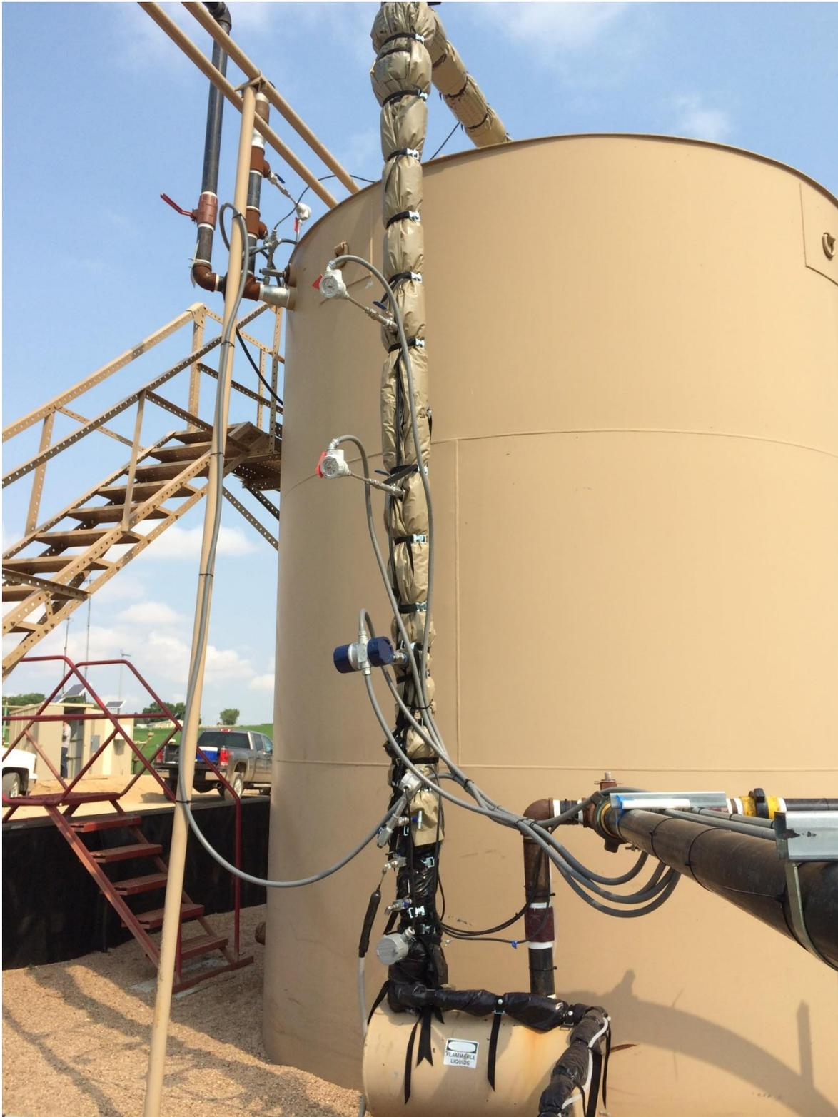
Figure IV.3-5. Condensate Storage Tanks with three gas flowmeters in insulated and heat-traced tank-to-burner pipeline. Gas sample collection port above knockout drum.
